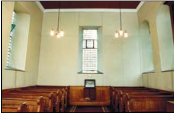
The rear of the chapel in 1994 before the door to the kitchen area was created. Note the false ceiling which was removed and the window which was reduced in size to make space for the new door
