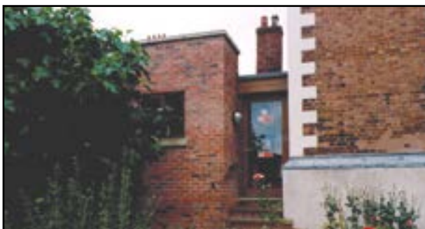
The new kitchen and toilets built in 1997
