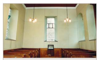
The rear of the chapel in 1994 before the door to the kitchen area was created. Note the false ceiling which was removed and the window which was reduced in size to make space for the new door
