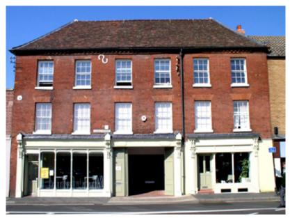
Extensive structural repairs and strengthening works were required to stabilise existing walls and floors that were discovered to be in a dangerous condition. The top hung casement windows have been replaced with vertical sliding sash windows.
